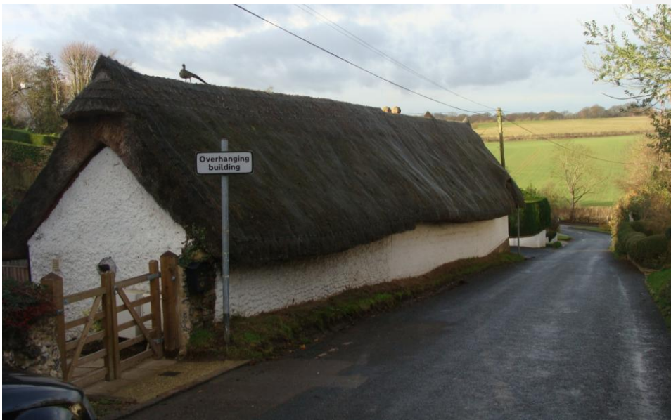
Picture 7 – Thatched building with clay lump walls at Ford Hill. It survives as an obsolete form of building construction of great interest.
