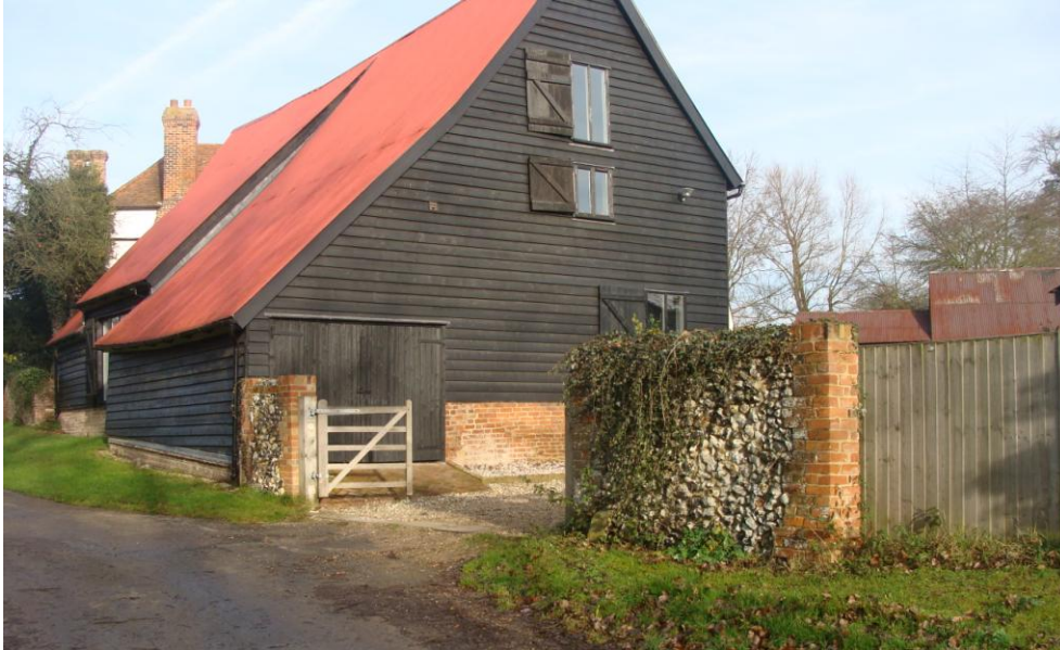
Picture 19 – within the parish there are numbers of roofs with replacement corrugated iron, some of which would originally have been thatched. This one, South Barn at Lower farm is in has been converted to ancillary residential use.
