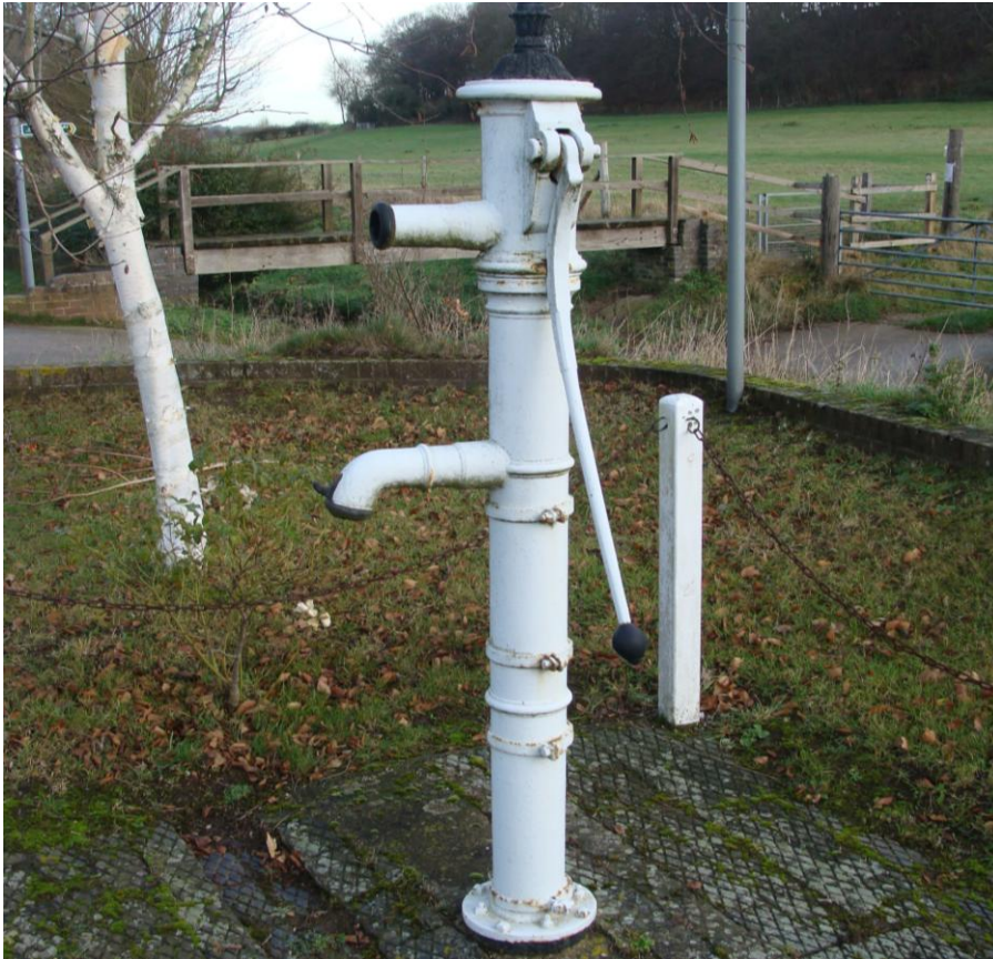
Picture 5 - A fine 19 th century pump of considerable artistic, social and technological interest. Several of the blue brick pavours need re-setting.
